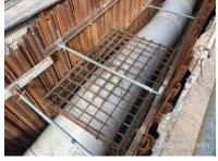
Construction of base slab of service reservoir
